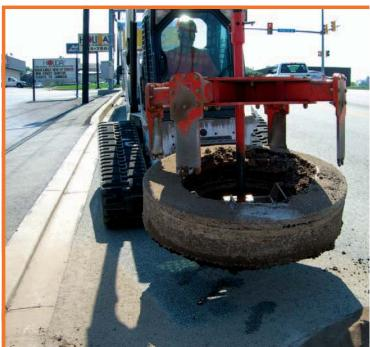
The device pulls the frame and road overcut in one operation.
