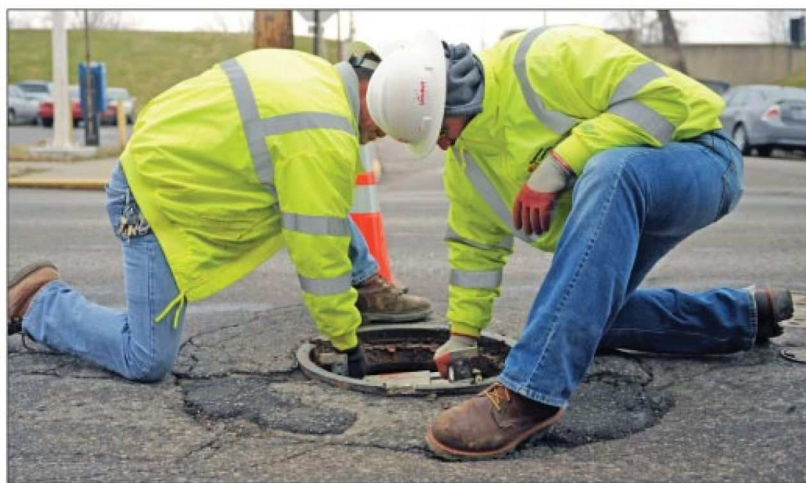
Upper photo: Phillip Ratts, left, and Nathan Pedigo tighten the speed plate of the Mr. Manhole system into place. The plate allows the cutting head to cut the old manhole loose from the street and remove it. Right photo: Ratts guides the cutter head over top the manhole. The head cuts into the pavement to release and then remove the old manhole.
