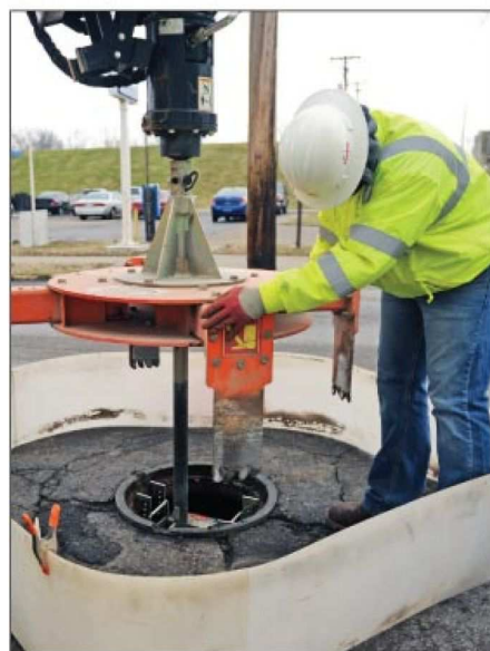
Upper photo: Phillip Ratts, left, and Nathan Pedigo tighten the speed plate of the Mr. Manhole system into place. The plate allows the cutting head to cut the old manhole loose from the street and remove it. Right photo: Ratts guides the cutter head over top the manhole. The head cuts into the pavement to release and then remove the old manhole.
