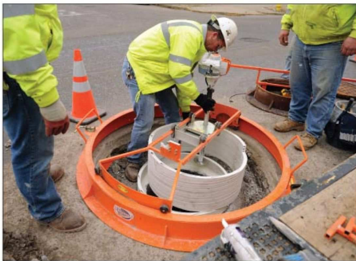
Phillip Ratts guides a manhole ring saw around the pipe to get a straight cut.
