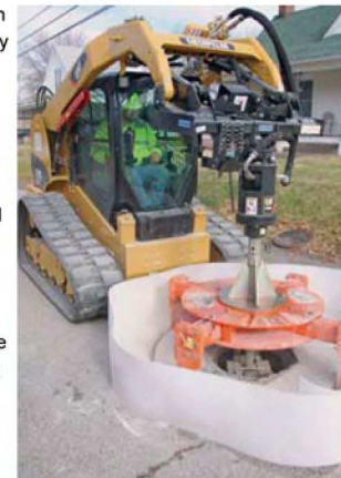
A Mr. Manhole cutter extractor, attached to a Caterpillar 279C compact track loader equipped with a Cat A26B high-flow auger drive unit, cuts through pavement in Hardinsburg, KY.
