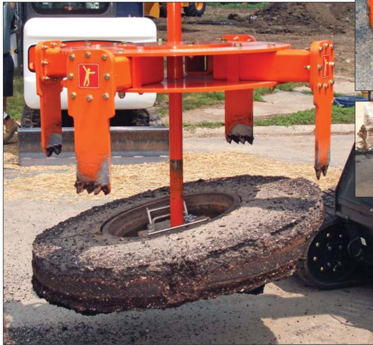
The operator lifts the circular segment of asphalt surrounding the manhole ring and moves it out of the way of the manhole area.
