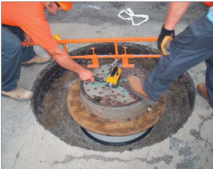
The ring is carried using a special tool and lowered onto the PVC liner. Then the manhole lid is put back in place.
