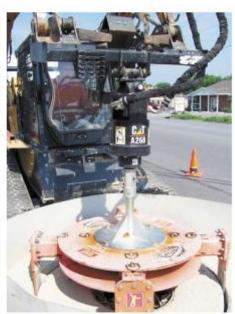
Rodney Brenneman with Brenneman Excavating, a certified Mr. Manhole installer, cut out the casting around the old manhole cover prior to installation of the new product. Concrete will be poured later and the new, smooth manhole will be installed.
