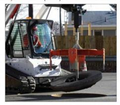
uses a plastic, stay-in-place form to prevent water and gas from deteriorating the cast-in-place, epoxy-coated, re-rod, reinforced concrete collar. The attachment works off an augerdrive to spin and cut through asphalt and concrete, removing the manhole casting and road over cut in just minutes. The tool works best on a unit with at least 20 gpm of flow and any auger drive will work (no special controls or hydraulic circuits are needed).
